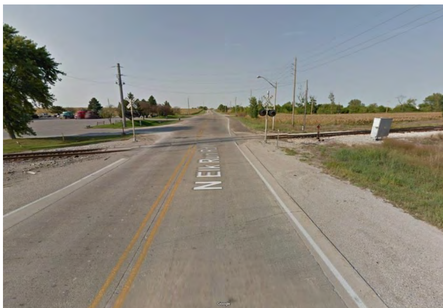
FIGURE 7: Google image of the UP Railroad Crossing of North Elk Run Road.
