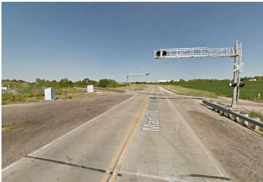
FIGURE 9: Google image of the UP Railroad Crossing of Martin Luther King Jr. Drive.
